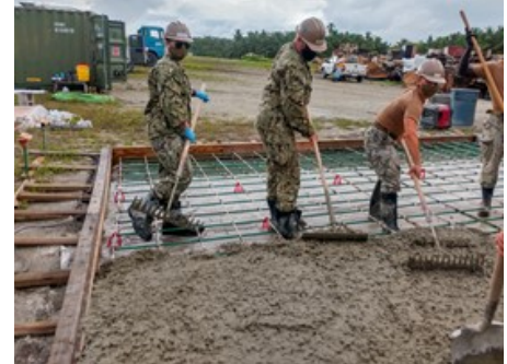
Seabees assigned to U.S. Naval Mobile Construction Battalion (NMCB) 3 place concrete at a construction site in Diego Garcia.
